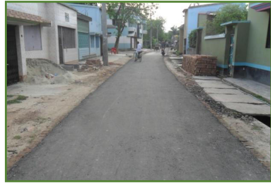
R13- Completed Pourashava road,
