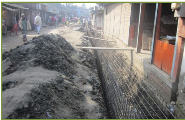
Construction of drain, Muktagacha
