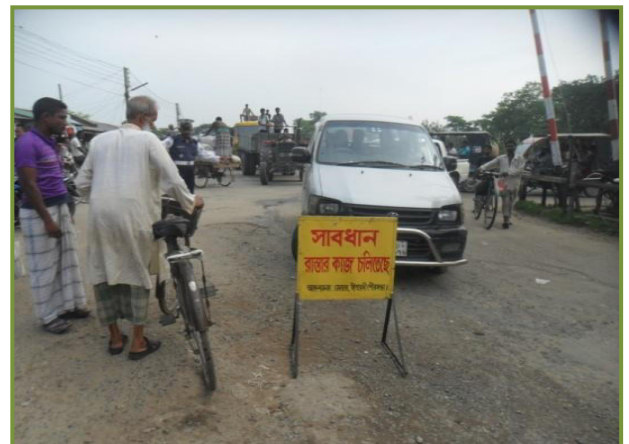
Indicating signboard at construction site, Ishwardi
